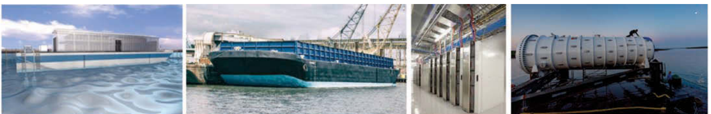
Figure 4. Nautilus Data Barges Ahead With Floating and Microsoft Underwater Data Center (1st from right)
